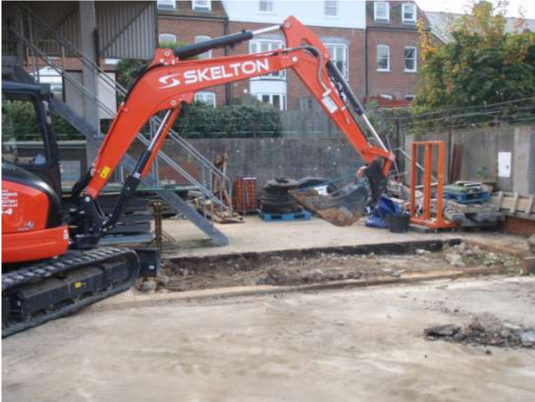
Plate 14. Trench D (looking south west)
